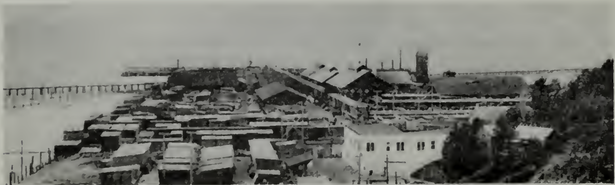
Steam Turbo Generating Plant of Hammond Lumber Company near Astoria - 1910
